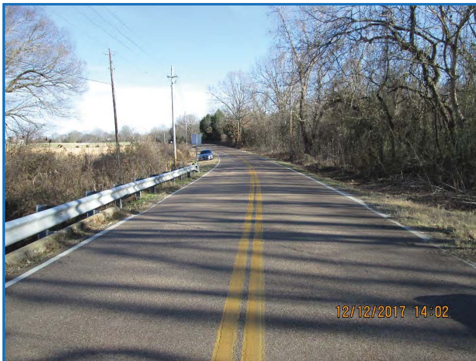
Looking east standing near middle of bridge
