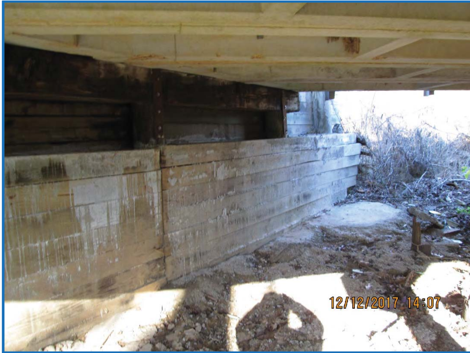
Looking at west abutment standing under bridge
