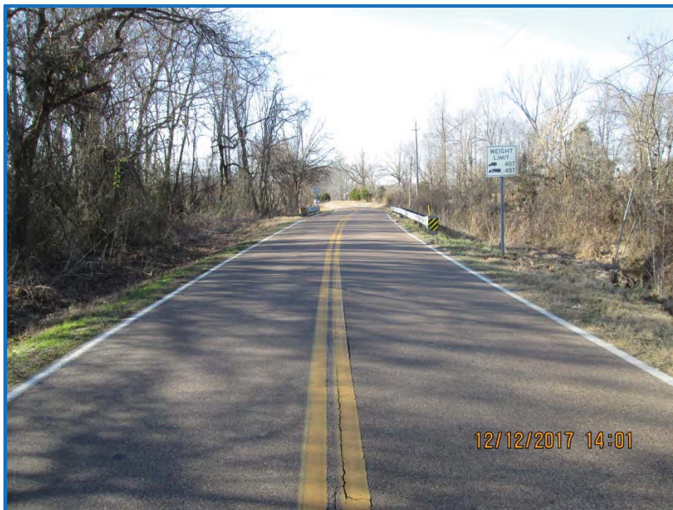
Looking west across bridge
