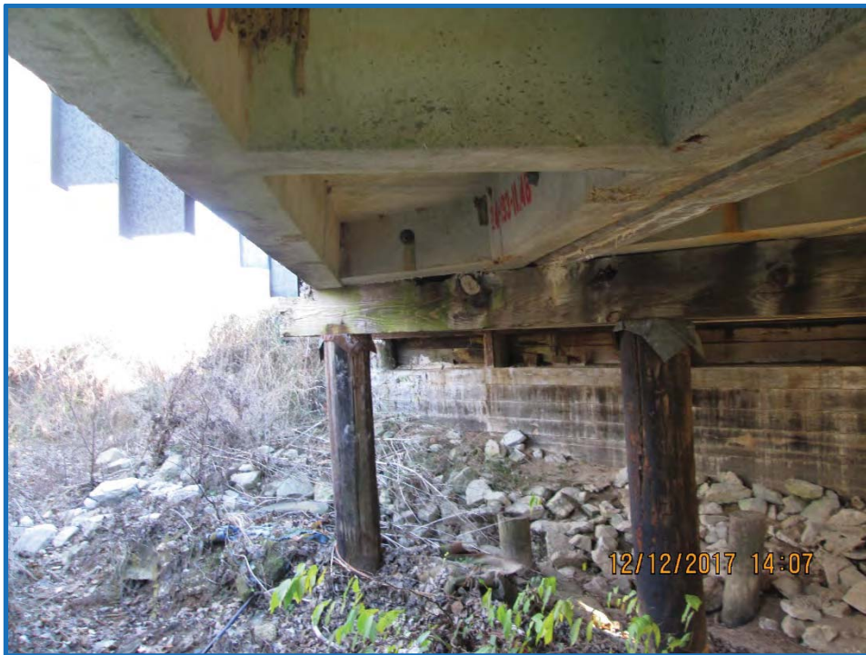
Looking at center pier and east abutment standing under bridge
