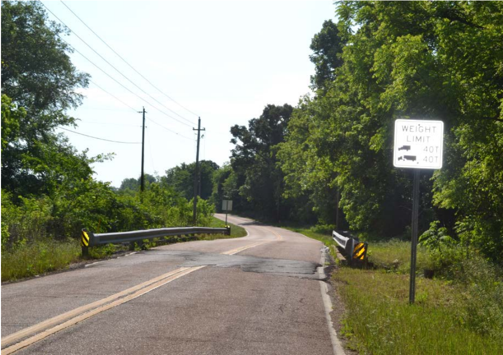
View east along SR-193 toward the bridge.
