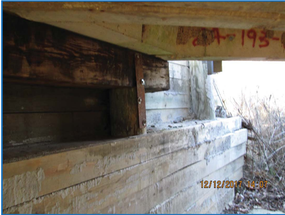
Looking at west abutment standing under bridge
